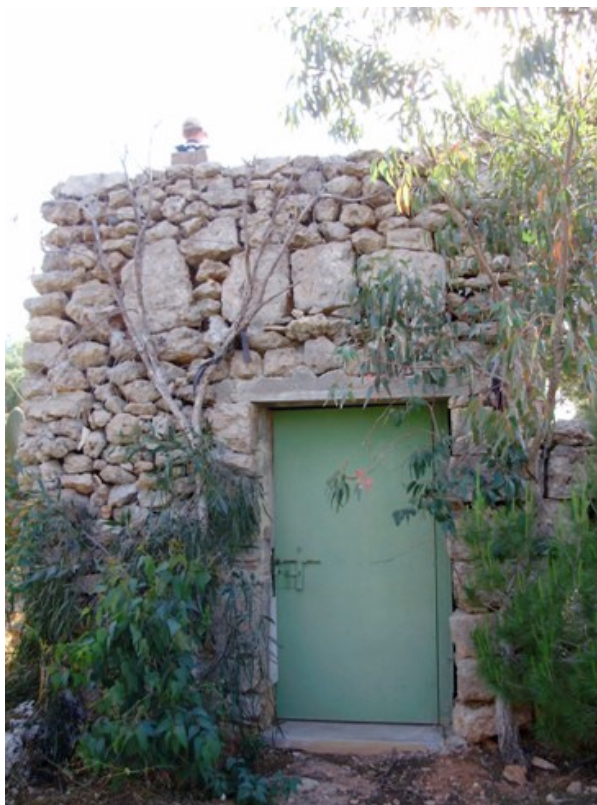
Images 1 & 2. Some of the illegally built hunting hides in Mizieb consist of two story concrete structures.
